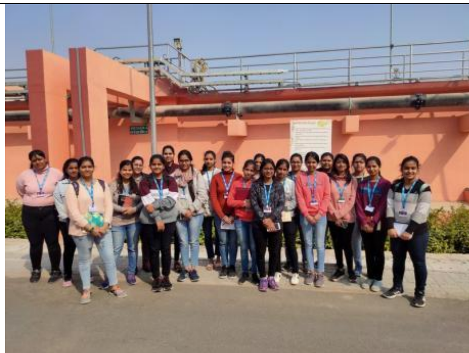
Visit to RIICO Sewage Treatment Plant (STP), Jaipur
